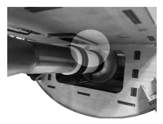
7. Use a rotary tool to make a small relief cut for the header in the former shown.
